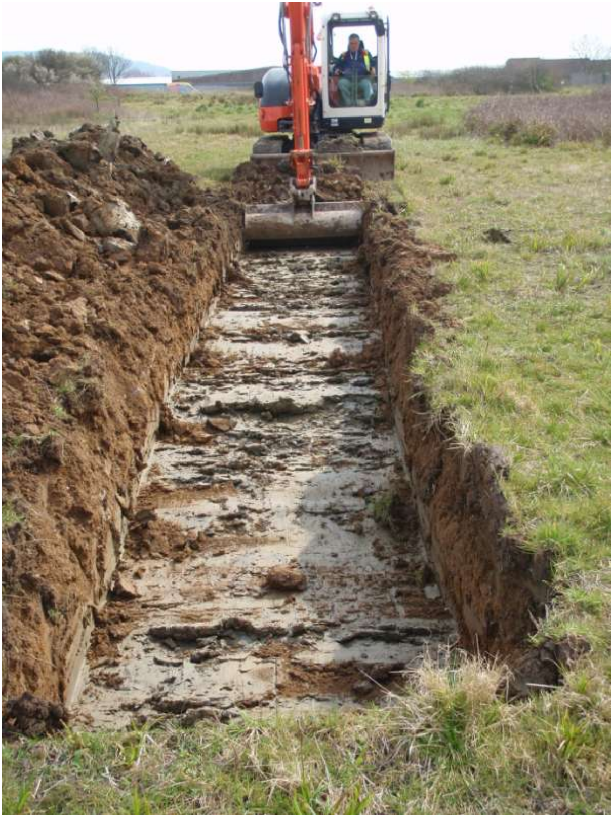
Plate 3 – Trench 2 (looking SE)
