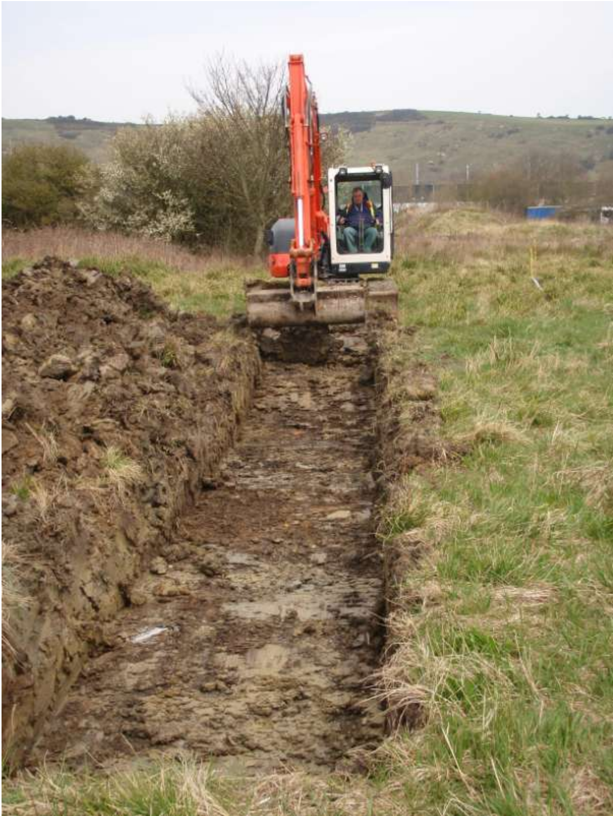
Plate 4 – Trench 3 showing quarry backfill (looking N)
